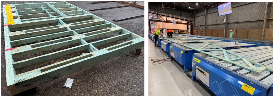
Figure 5: Timber wall frame (L). Timber truss being assembled (R)
