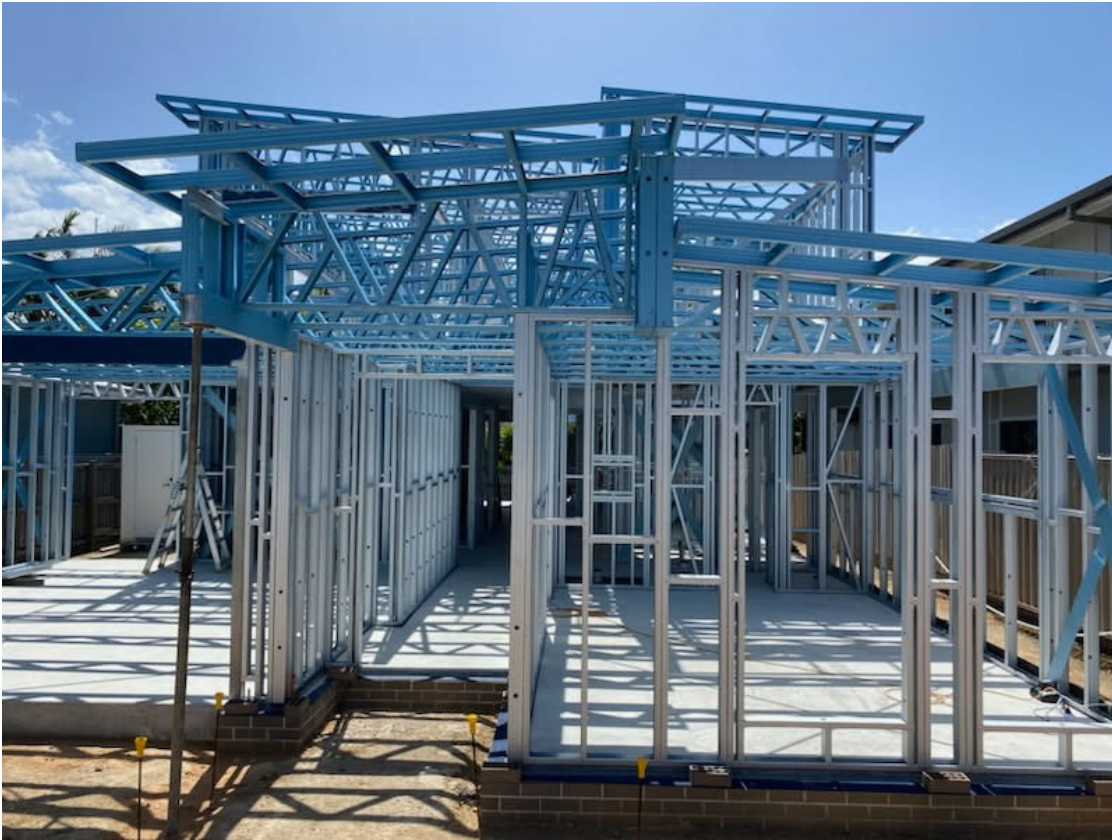
Figure 6: Steel house frame
